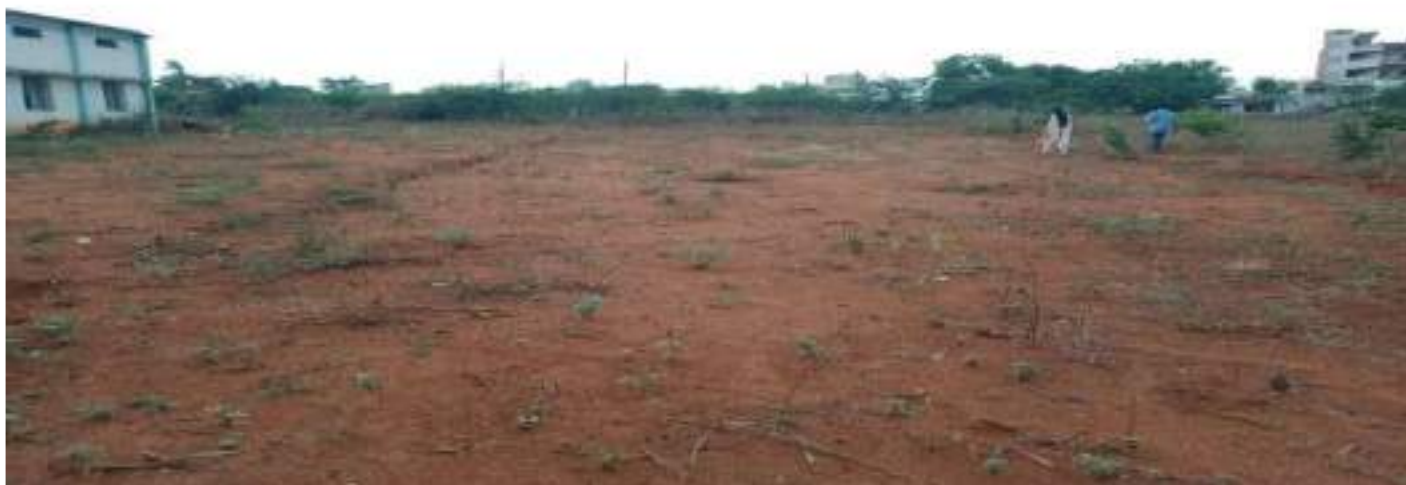
Preparation of land
